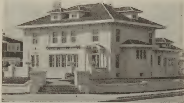
HOUSE OF JOHN L. POWELL, WICHITA, KANSAS HERMAN J. STROEH, ARCHITECT STUCCO ON INTERLOCKING TILE.
